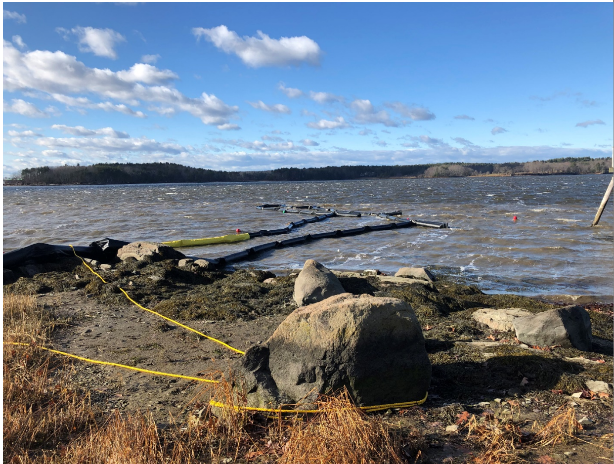
Mackworth Env barrier after breaking free. The barrier was drifting toward the Beswick dock to the right. Mackworth secured the barrier in place out of the way of the diver barges.
