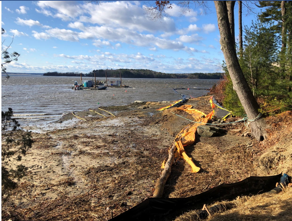
View from Gundalow Landing site, looking at Adams Point, with two dive barges spudded in place. Mackworth Env turbidity barrier failed by breaking free of its southern anchors and drifting to the north.
